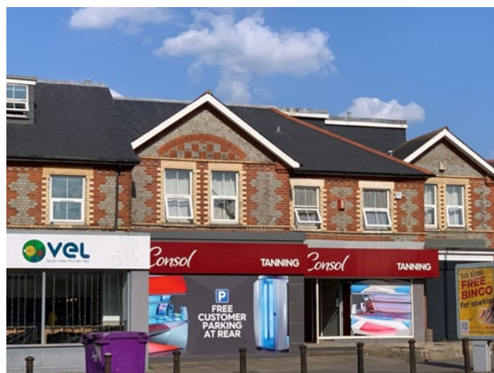
Film covered shop windows at 79 Whitley Street
